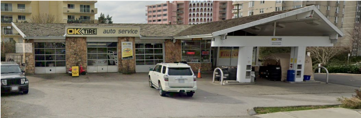
Figure 3: Image of the north (front) elevation of 2196 Marine Drive as it looks today
