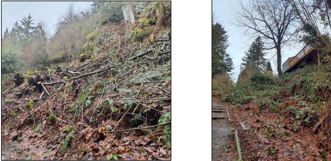
Figure 1: Examples of slashed material on a transmission line right of way (left) and unmanaged vegetation on a residential distribution line right of way (right).
