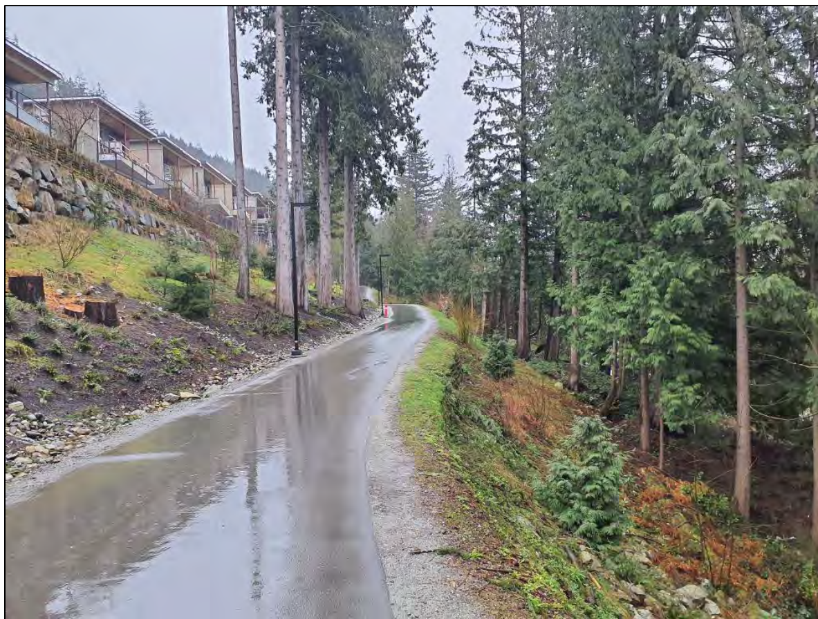
Figure 9. Example of proactive vegetation management and emergency access in Area 6: 1) conifer trees removed or pruned on the high side and deciduous shrubs planted; 2) deadfall removed, trees spaced and pruned on the low side; 3) paved access to the interface area downslope of structures.
