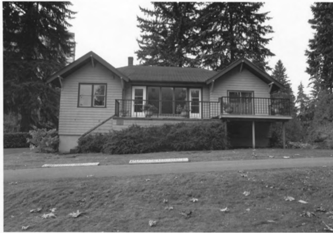
Original Main House—demolished
