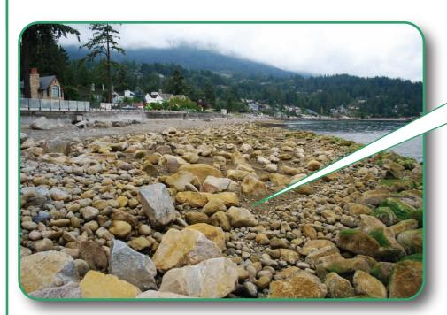
Construction of a buried berm and elevation of the upper shore, using recycled and native beach materials, help to trap and stabilize fine sediments.
