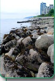
Riprap from the seawall was repositioned along the shoreline to create wave trips and tombolas. Wave trips disrupt wave energy on the lower shore, providing
