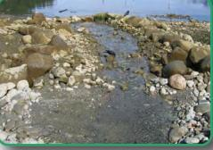
Large boulders lining the culvert direct the flow, reducing the speed and erosive force of the stream during high flow events. The resulting channel can be used by various species of birds for preening and drinking. Habitat boulders at the end of the channel disseminate fresh water across the lower shore and provide valuable habitat for algae and invertebrates such as mussels which benefit from access to fresh water.
