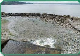
Strips of boulders along the channel deflect the stream along the beach which slows the flow, reduces erosion and causes sediments carried in the stream to be deposited on midshore. Groups of boulders also act as tombolas, guiding and trapping sediments carried to the shore by waves and currents.
