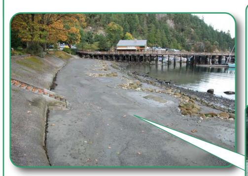
A cobble and boulder bench was built along the lower shore to protect the beach by tripping waves and dispersing their energy. A series of crescent shaped cobble and boulder berms elevate and stabilise the upper shore, which was thickened with fine sediments. By increasing the gradient and roughening the lower shore, the beach was returned to a natural state to protect and replenish the shoreline.
