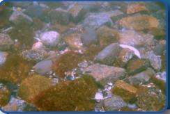
The existing hard-faced wave defense measures were not suitable for colonization by most algae and invertebrates. The riprap berm, built to reduce wave impacts and effects of prop-wash on the site, provided an opportunity to create subtidal and intertidal habitat for algae, invertebrates and fishes
