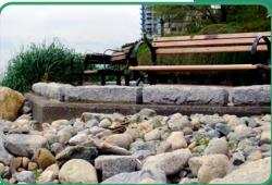
Using boulders and salt marsh to elevate the upper shore and create a more natural, sloping shoreline, closes the gap between the beach and the Seawalk. The wave trips, drift sills and tombolas will continue to trap sediments and increase the beach profile, closing the physical gap between the Seawalk and the beach and improving public access to the shoreline.
