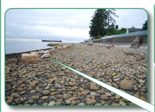
A row of large boulders along the lower edge of the berm act as wave trips, disrupting wave energy before they reach the upper shore. The elevated and sloping upper shore provides greater resistence to waves and a second line of wave protection in front of the sea wall on the upper shore, provide extra reinforcement during high water and extreme weather events.
