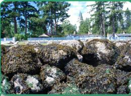
Large boulders used to stabilize sediments also function as fish habitat by providing space for algae and invertebrates to colonize, creating shelter and feeding grounds for fish. Rebuilding the upper shore encourages the re-growth of the riparian zone and expansion of the existing dune grass patches.
