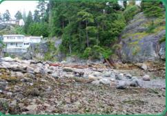
Strategically placed boulders on the lower shore 'trip' incoming waves, causing them to break and lose energy before they reach the upper shore. By doing this they protect the upper shore and upland from damage and erosion by waves and debris. Wave trips provide long term protection and are ecologically sound as they provide habitat for algae and invertebrates.
