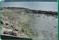
Strips of boulders direct the channel along the shore, instead of allowing it to flow straight out to sea, causing sediments to be deposited on the beach. Strategically positioned boulders guide and trap sediments in areas vulnerable to erosion and also act as 'wave trips', tripping waves before they reach the upper shore reducing their erosional force.
