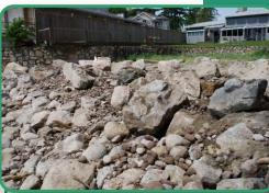
The upper shore was elevated using large woody debris, covered with fine sediments and planted with dune grass to create a natural salt marsh. The complex root system of dune grass helps to stabilise fine sediments. The profile of the midshore was raised using riprap and cobble to create a naturally sloping shoreline which will provide more resistance to waves and protect the upper shore and salt marsh habitat.
