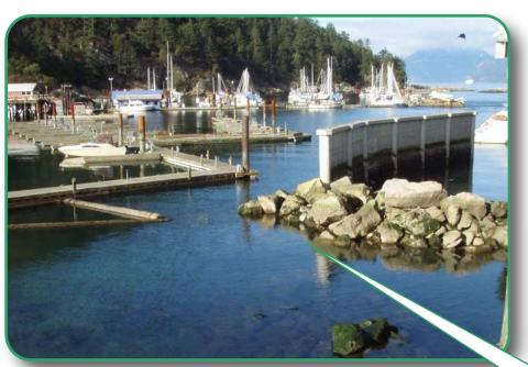
Construction of a rock berm at the shoreward end of the wave deflector improves shoreline protection by disrupting wave energy. The rock berm acts like a natural reef, protecting the shore from erosive waves and propeller wash while providing habitat for algae, invertebrates and fish. The reef will become more effective wave protection as kelp and broad-leaf algae grow.
