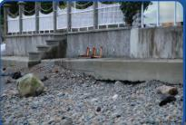
Wave erosion is typically amplified by urban developments such as hard-faced seawalls, as they reflect waves back down the beach instead of disrupting them. Heavy erosion had undercut sections of the seawall at 27th street making the wall itself vulnerable to damage. Sustainable and effective shoreline protection can be created by using measures that work with coastal processes instead of combatting them.
