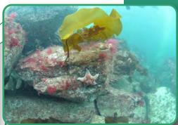
The riprap berm wave protection was extended to create an algae bench. The large boulders provided a stable attachment point for broad-leafed algae, such as kelp. Gaps between the boulders and the algae itself create shelter, feeding and spawning grounds for many invertebrates and fishes. Kelp beds are key features of a healthy marine ecosystem and support productive fisheries.
