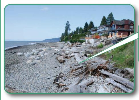
Strategically placed boulders create tombolas and drift sills which guide and trap sediments on the upper shore, continuously replenishing the beach.
