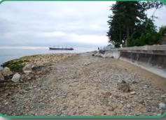
Large boulders guide and trap fine sediments as they are carried along the beach by longshore drift. By elevating the upper shore and raising the beach profile, erosion is prevented and the newly trapped sediments are protected. As they work with natural coastal processes, these methods can provide a long term solution to erosion and help build and maintain a natural upper shore for years to come.
