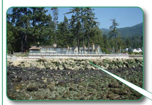
Large boulder riprap was used to construct a berm along the mid-intertidal zone to roughening the lower shore and disrupt waves before they reached the upper shore. The berm was then backfilled with natural and reclaimed materials raising the upper shore and creating a gentle gradient, increasing the resistance to waves travelling up the beach.
