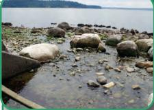
Large boulders placed along the shore direct the stream channel and ensure that it does not get eroded by waves. Boulders in the creek increase the complexity of the channels, creating riffle pools and meanders which provide a more diverse habitat for fishes and invertebrates, providing shelter and feeding opportunities for migrating salmon.
