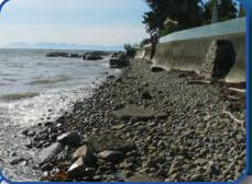
Waves that strike the hard-faced sea wall are reflected back down the beach gathering momentum with gravity and carrying away fine sediments to deeper waters. A natural irregular and rocky shore line disrupts waves on the lower shore, preventing waves from heavily impacting the upper shore and the overtopping the sea wall.
