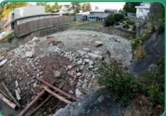
Riprap drift sills were installed along the mid and lower shore to protect the salt marsh through its first winter storms. The following spring the drift sills were dismantled and the rip rap was spread along the mid shore and covered with cobble to raise the profile of the beach, improving the natural wave resistence. Large riprap wave trips provide further protection and intertidal habitat.
