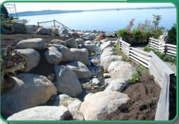
The ground flow was brought to the surface (daylighted) through a channel. The new creek was created with riffle pools, meanders, and shelter for insects and fishes. The new riparian zone also creates important habitat for insects and birds. Insects and their larvae, plant material and seeds are an important food source for juvenile fishes along the coast.
