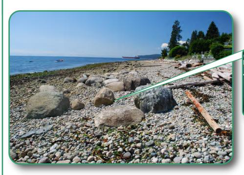
Strategically placed patches of large boulders and logs guide and trap fine sediments on the upper shore as they are carried in by waves. Drift sills positioned at the end of the new creek
