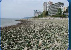
A low profile, loose cobble beach with a hard-faced concrete sea wall is exposed to increased erosion. Waves that reach the sea wall are reflected back down the beach full strength, where they gain momentum with gravity and sweep sediments out to deeper water. Erosion would be greatly reduced by disrupting vaves on the lower shore
