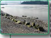
Large boulder 'wave trips' were placed along the shore line. As waves travel inshore they strike the
