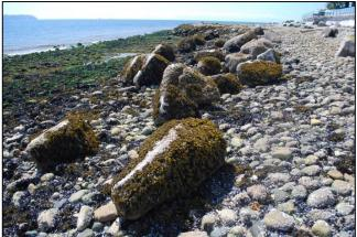
Additional large boulders were partially buried along the upper shore. In front of the sea wall, to stabilize fine sediments and provide improved wave protection by 'tripping' waves and diffusing wave energy before they meet the sea wall. Post-construction surveys have recorded increased sediment retention on the upper shore and almost complete coverage of the intertidal habitat boulders by invertebrates and algae.
