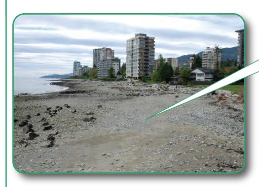
Boulders placed along the midshore guide and trap sediments carried by currents and waves, replenishing and rebuilding the beach gradually but over a long term basis.
