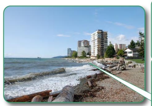
Large woody debris and boulders were used to create a more natural sloping, irregular shoreline which diffuses, rather than reflects, wave energy thereby reducing beach erosion. Using natural materials and working with coastal processes to restore the shoreline provides long-term benefits and sustainability while creating valuable natural habitat for marine species.
