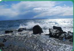
Large boulder 'wave trips' were positioned along lower shore. Waves travelling in-shore strike the wave trips and then break, diffusing their energy. Wave trips act like a natural rocky shore line, reducing the power of waves before they reach the upper shore, they provide a long term solution to erosion and create habitat for many intertidal species.
