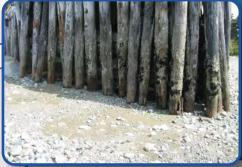
Soft wave protection, such as wave trips, tombolas and berms 'roughen' the shoreline, returning it to a more natural state. Shoreline roughening works with coastal processes to provide long term protection from waves and prevention of erosion, creating a self-sustaining shoreline.
