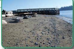
As the beach profile increases it further stabilises the sediments, interrupts the historical cycle of erosion and provides more protection to shoreline developments.
