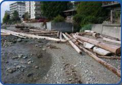
A hard-faced, vertical sea wall may provide some protection for shore line developments, but it can actually contribute to beach erosion in the long term as, instead of disrupting wave energy, it reflects waves full-force back down the beach. Returning the shoreline to a more natural state provides sustainable and improved protection.
