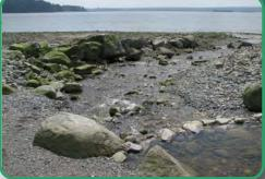
The channel was deepened and boulders along the banks prevent erosion. Logs and boulders create riffle pools, meanders and shelter providing important habitat for fishes, especially salmon. From 2003- 2005 no salmon were reported in Lawson Creek; the year following the project the West Vancouver Streamkeepers Society recorded 51 salmon.
