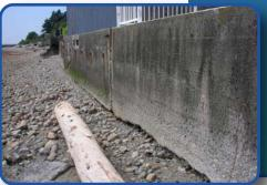
Certain areas of the beach between 15th Street and Ambleside have experienced heavy erosion of fine sediments leaving a pebble and cobble beach. Hard-faced concrete seawalls protecting shoreline developments are themselves compromised and damaged by wave action and erosion.
