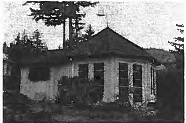
FINGUENEISEL SUMMER HOUSE 6043 GLENEAGLES DRIVE Theo Korner, Architect, 1938
