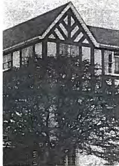
'HOLLYBURN MANOR' 565 17TH STREET 1940, DEMOLISHED 1988
