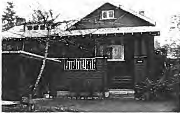
HODGSON HOUSE 2355 MARINE DRIVE Hugh Hodgson, Architect, 1913
