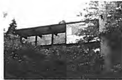
KENNEDY HOUSE 3351 CRAIG END ROAD Sharp & Thompson, Berwick, Pratt, Architects, 1954 Designed by Roy Jessiman; an excellent example of early post and beam construction.
