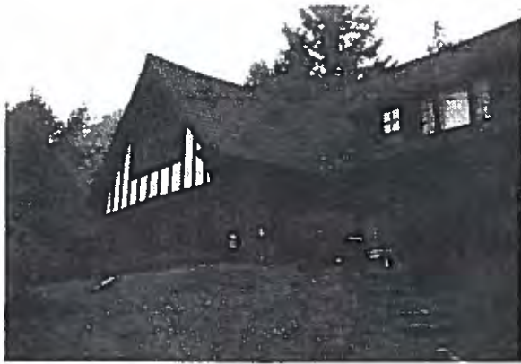
GEORGE MEREDITH PUGH HOUSE 2165 GISBY STREET C.B.K. Van Norman, Architect 1936
