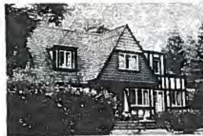
PALMER HOUSE 2979 MATHERS AVENUE 1938, DEMOLISHED 1989
