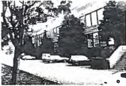
PAULINE JOHNSON SCHOOL 1150 22ND STREET Hugh A. Hodgson, Architect 1921 and 1922-1923 ALTERATIONS 1992 Heritage Achievement Award, 1995
