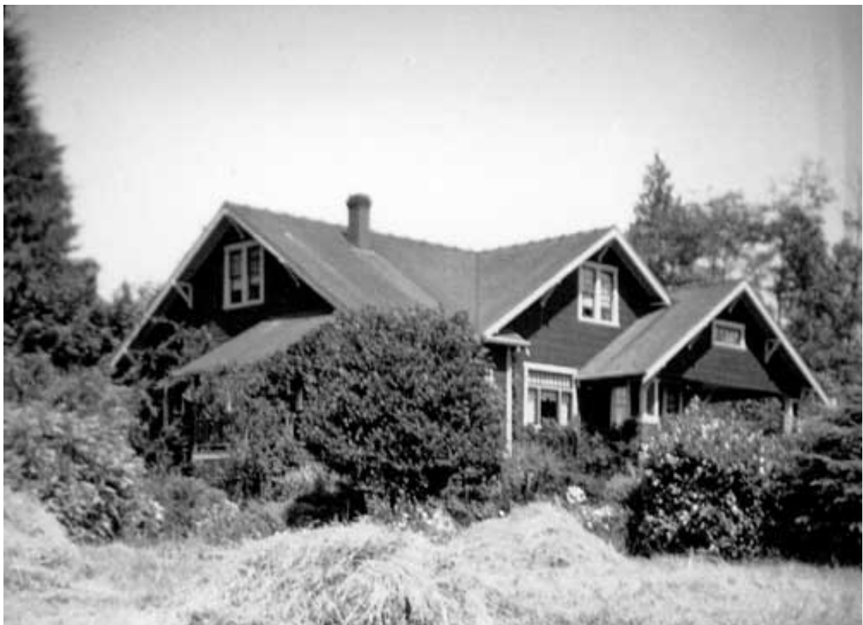
Rush House and surrounding hay field, between 1923 and 1929, West Vancouver Archives 13265.WVA.PHO
