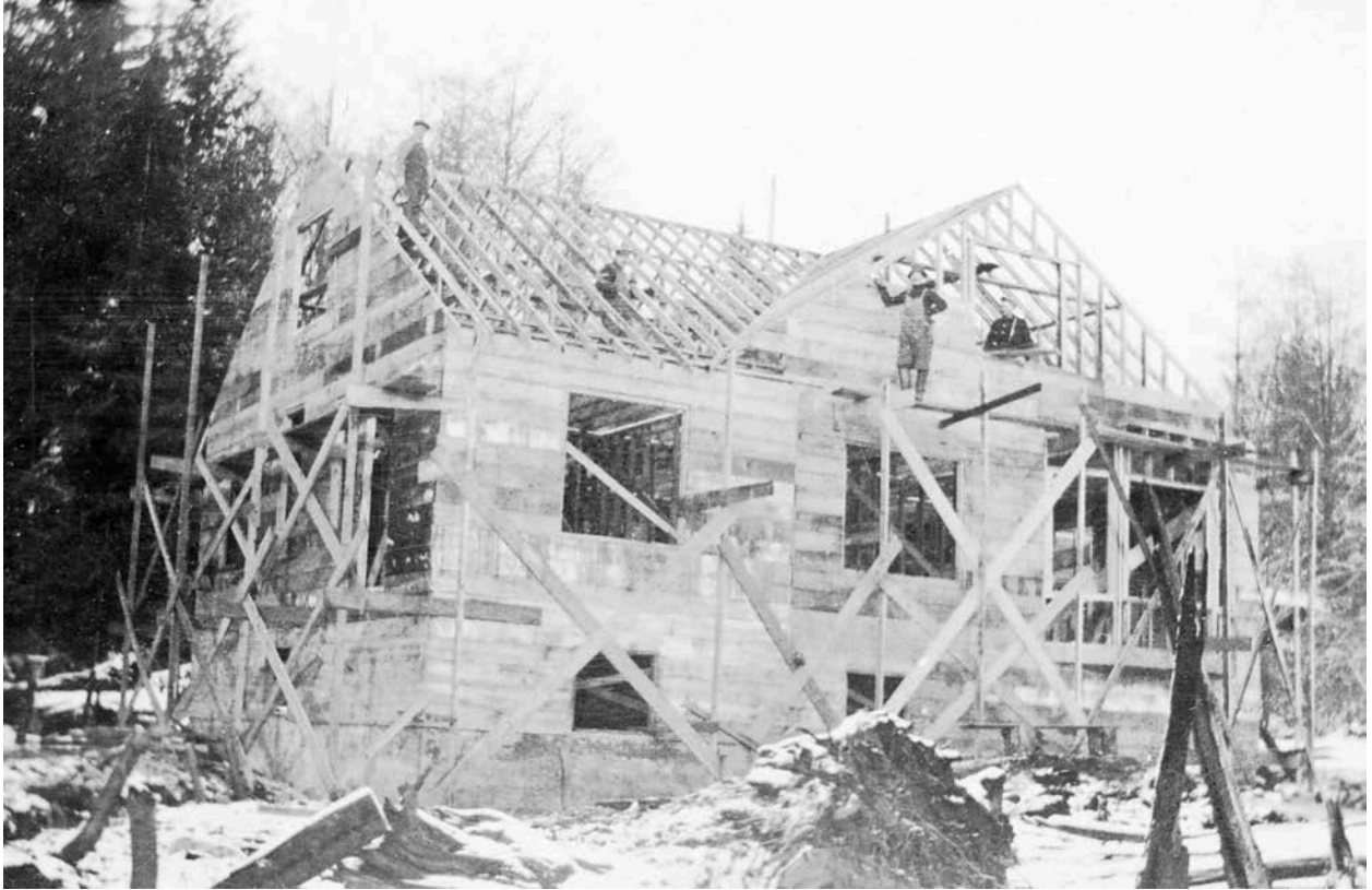
Rush House under construction, 1923, West Vancouver Archives 3267.WVA.PHO
