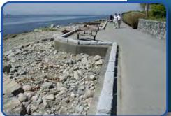
Replacing the existing hard-faced sea wall with softer shoreline protection measures will improve the physical and aesthetic accessibility of the shoreline to the public. By using natural coastal processes to trap sediments on the upper shore the gap between the seawalk and beach will be reduced, reconnecting the Seawalk with the foreshore.
