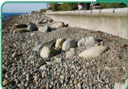
Wave trips, tombolas and riparian vegetation are used to create a self-sustaining shoreline. Wave trips along the lower shore break waves before they reach the upper shore, disrupting wave energy. Tombolas created along the beach guide and trap sediments that are carried by waves and currents, and the complex root systems of riparian plants help stabilize the upper shore.
