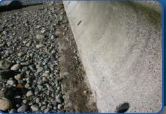
A low-profile, cobble beach with a hard-faced concrete sea wall offers little resistence to beach erosion. Waves hit the sea wall full force and are reflected instead of breaking. As they travel back to the ocean they carry sediment away from beach to deeper waters. Soft shoreline protection measures trap fine sediments on the beach while providing wave protection for the seawall.
